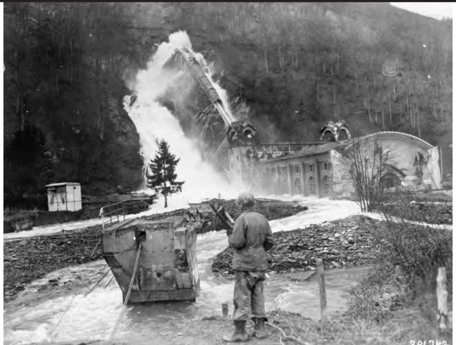
ABOVE: An American soldier watches torrents of water from the River Rur flow around the Heimbach hydro electric plant after the Schwammenauel Dam was breached in February 1945. OPPOSITE: A line of American troops crosses a bridge and marches through one of the many small villages that dot the Hürtgen region. The difficult hilly and forested terrain is very obvious in this photo, taken November 16, 1944.
