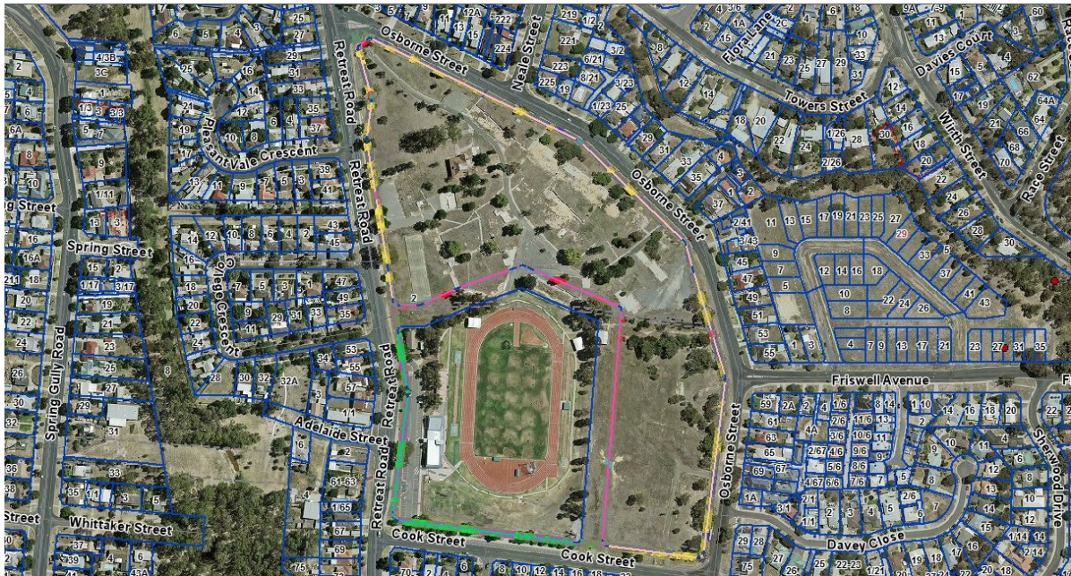
Figure 3: An aerial view of the subject site.
