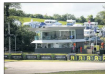
New control centre at Lydden
