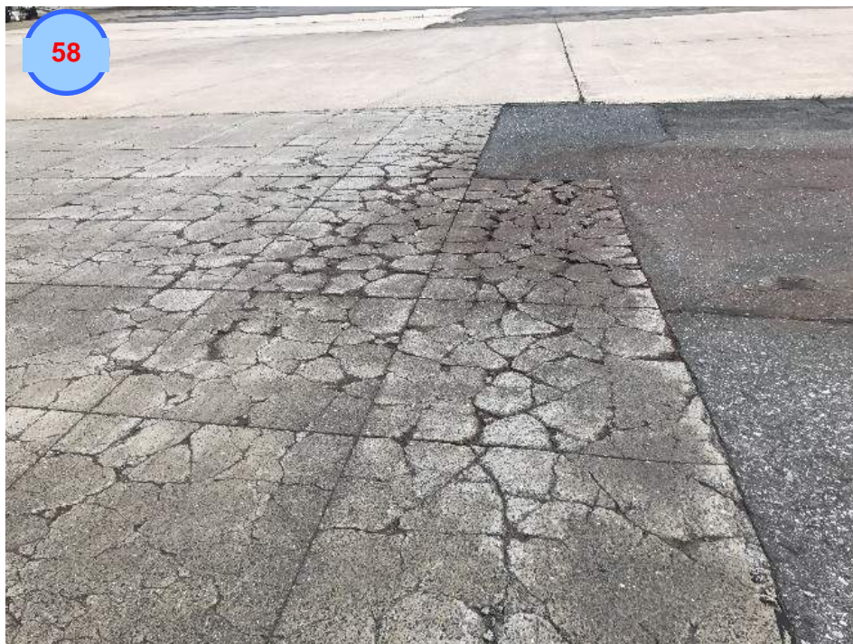
Shattered Slabs- East Section PCC
