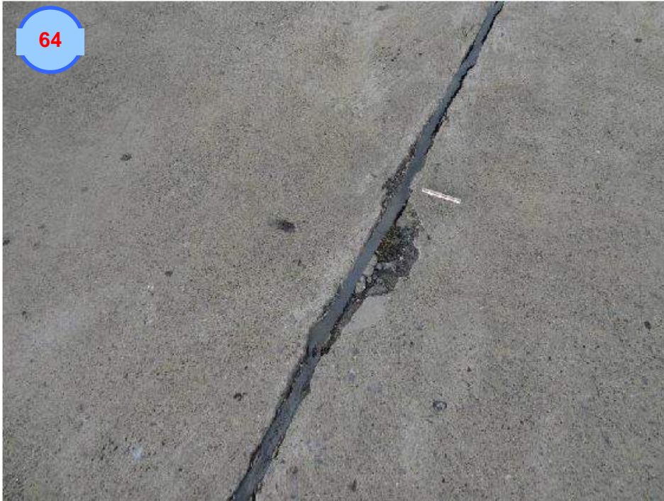
Joint Spalling
