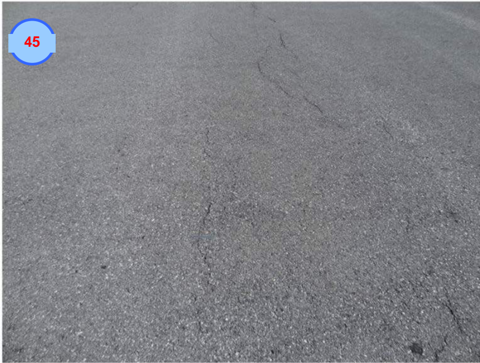
Weathering AC Section
