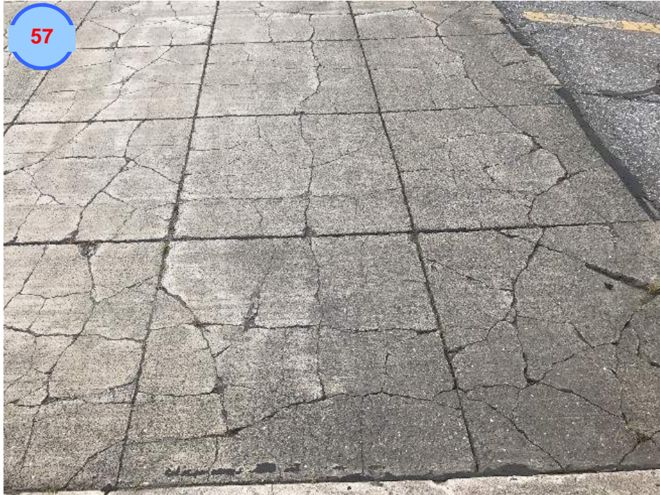
Shattered Slabs East Section-PCC
