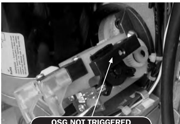
OSG NOT TRIGGERED OSG Regulator weight in level position
