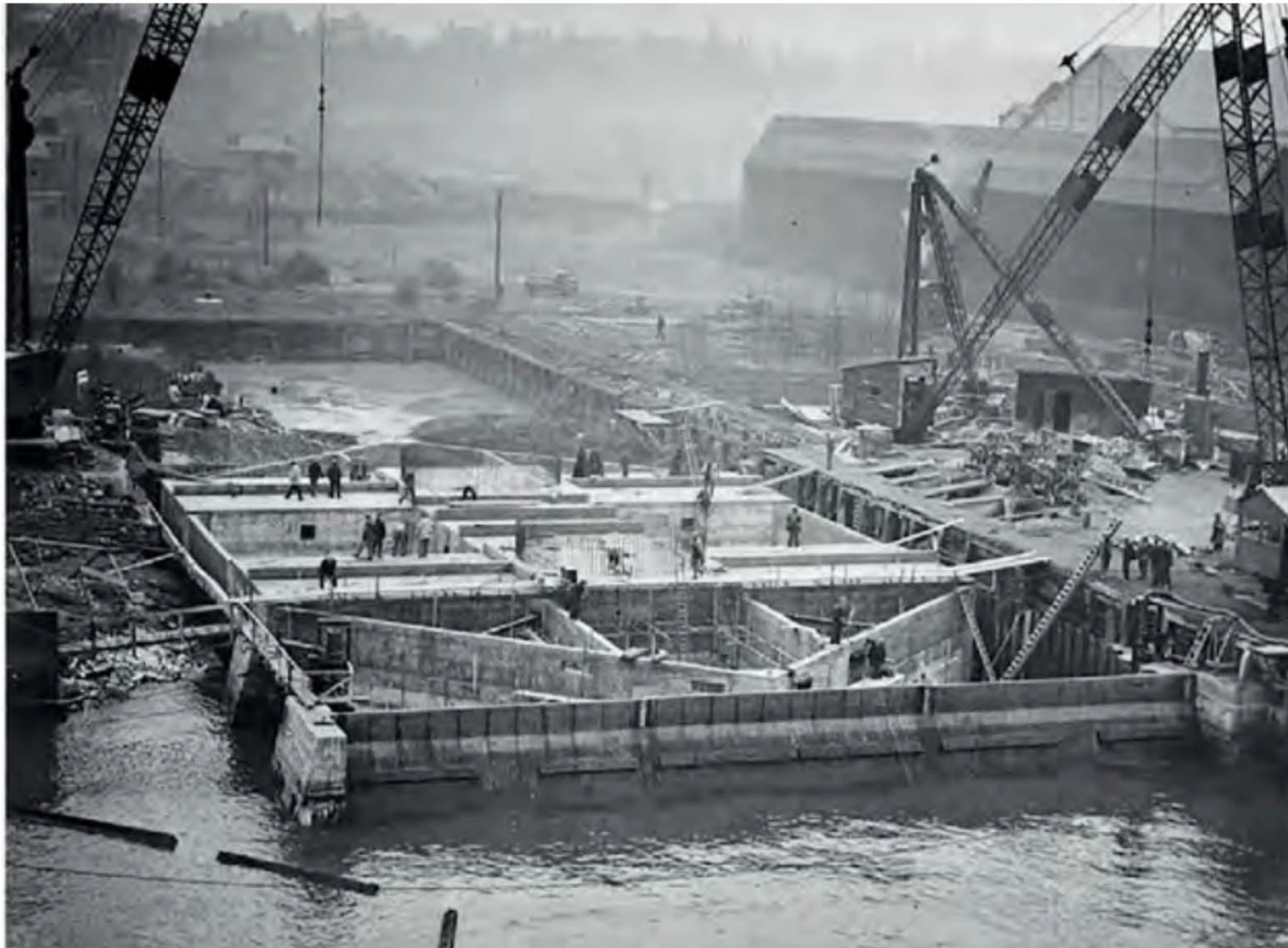
RIGHT A completed pontoon that will form the base of a sea fort to be used in the Thames Estuary c. late 1941/early 1942.
