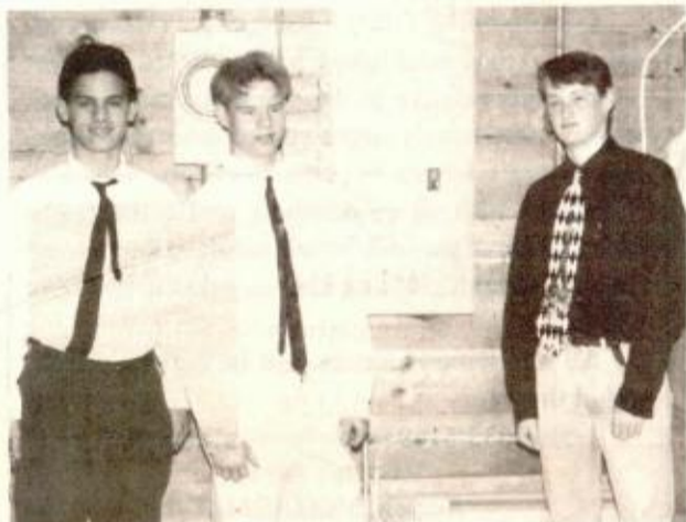
JUNIORS in the electrical lab at Don Bosco Technical High School in Boston are shown at a residential electrical panel. From the left are Eric M. Anoli of East Boston, Michael P. McGonagle of Charlestown and Michael Babcock of Brighton. The students are trained to be apprentice electricians or electrical helpers.
