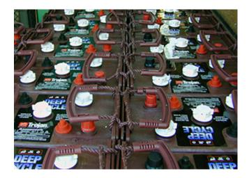
You can also apply a thin coating of petroleum jelly to the battery terminals for some extra protection.
