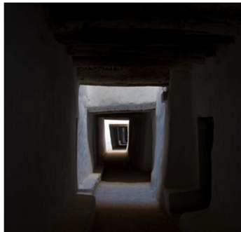
Picture 8. An interior view of a street shows the lighting the streets by the lighting and ventilation shafts
