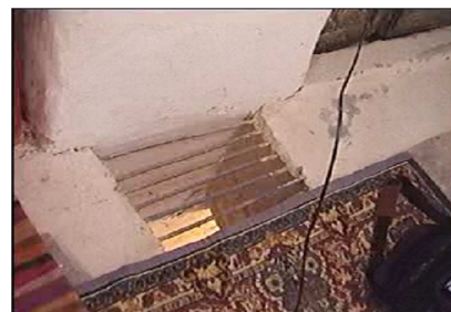
Picture 11. A view of the ventilation opening between the ground floor and the courtyard where the view was taken
