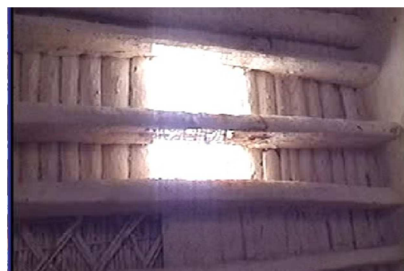
Picture 10. An interior view of the courtyard opening.
