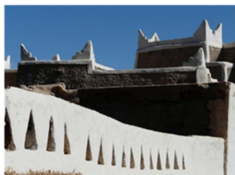
Picture 3. Side view shows the use of Malqaf in upper the houses
