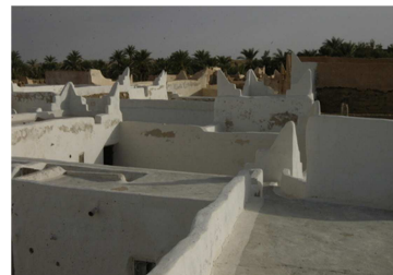
Picture 4. A view from the roofs shows the windcatchers on the kitchens' roofs
