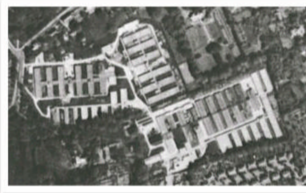
RAF Eastcote, pictured from the air in 1945. This government site was an outpost for Bletchley Park's codebreaking operations
