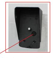
2. Mark a hole for the power and ethernet cable to run through. Remove the bracket, and then drill the holes. We recommend any holes you drill in your walls are sealed water tight. After threading the cables through.
