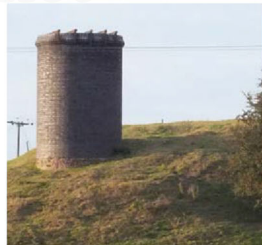
A Victorian aeration shaft on rising ground is the only clue to the hi-tech preparations going on below
