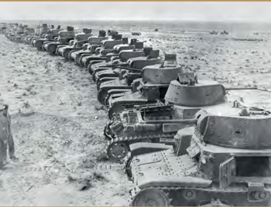
Captured Italian Carro Armato M13/40 medium tanks in Libya, North Africa, July 1941. It only had 30mm frontal armour on the rounded glacis. A two-pdr APCBC round could penetrate that armour at 1,000 yards. AWM/PD
