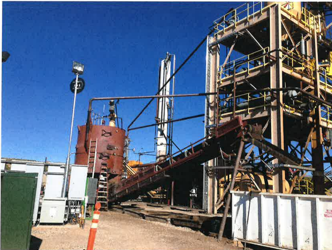
Pilot Bitumen Extraction Plant – Product Storage Tanks
