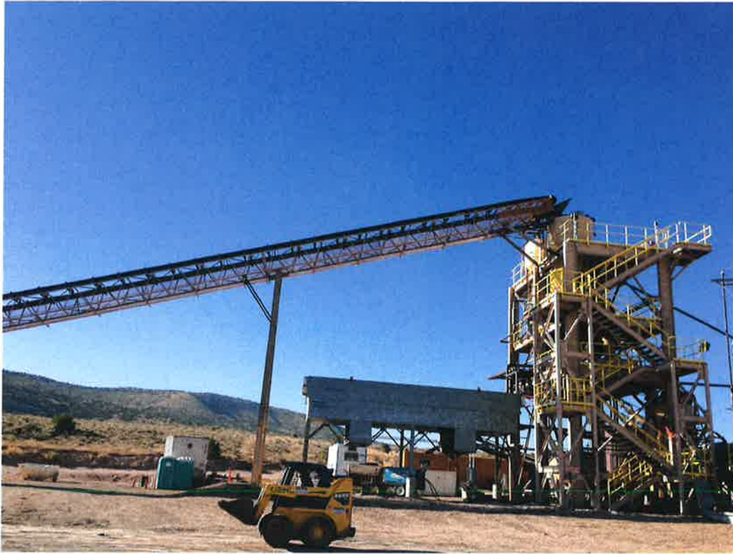
Pilot Bitumen Extraction Plant - Overview
