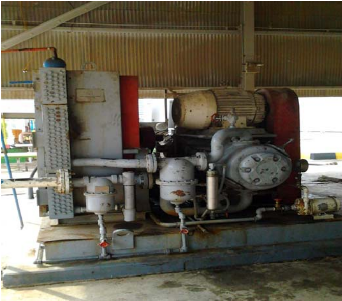
Electrical pump of fire fighting in desalination factory
