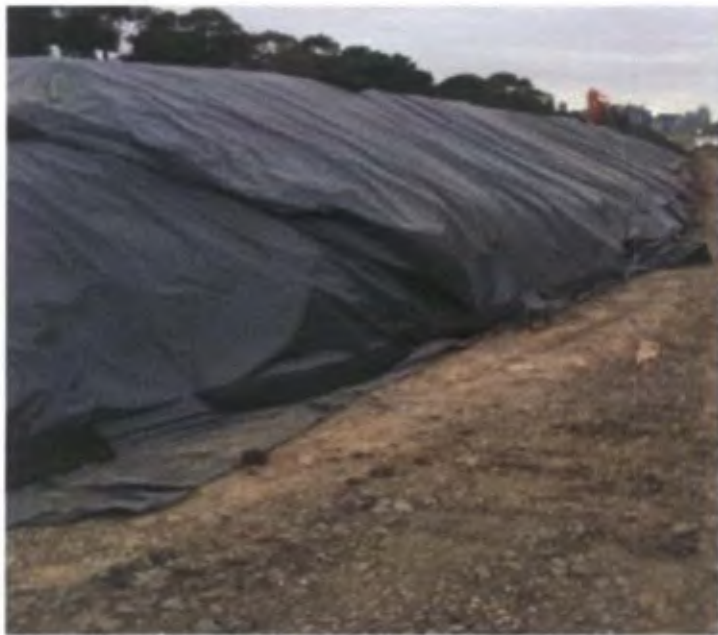
Stockpile on Footscray Road – Gate F02
