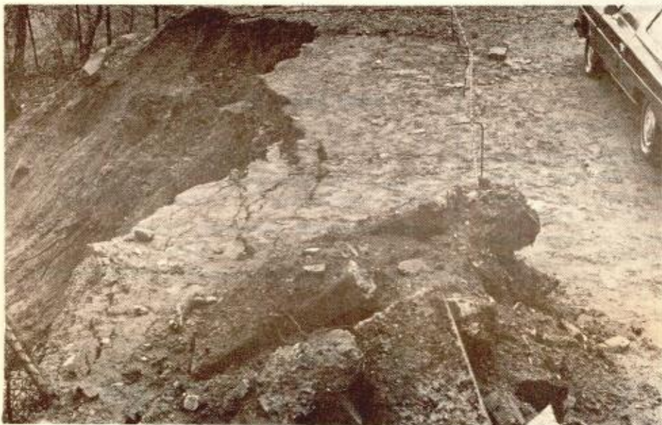
EROSION of the land to the rear of 21 North Mead Street following a mud slide on April 5 and 6. According to Patrick Murphy, attorney for the Murray family of that address, "the slide buried cement that had been
