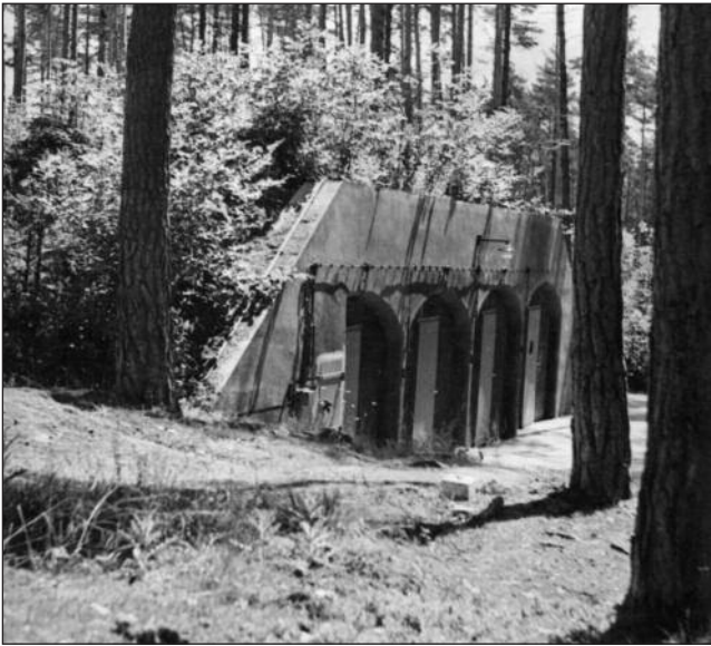
Left: Werk II included many buildings specially constructed for the safe handling of munitions, like this storage bunker with
