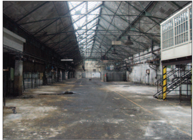
Today the whole factory stands empty and disused, the last industrial user having ceased production around the year 2000.
