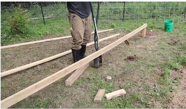
FIG 4. MIDDLE ANCHOR POST
