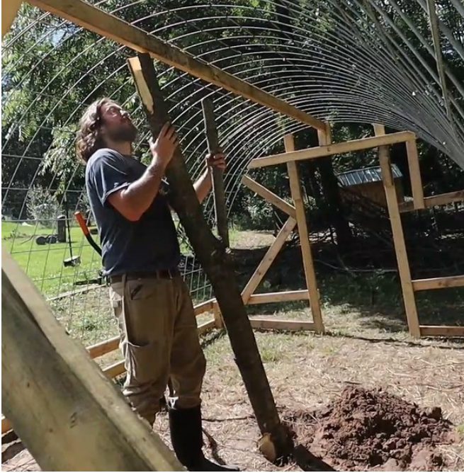
FIG 39. RIDGE BEAM SUPPORT
