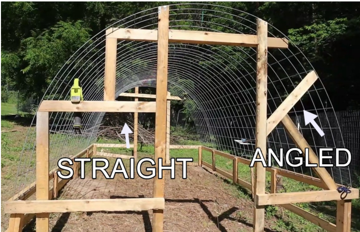
FIG 32. THE DIFFERENT BRACES SHOWN
