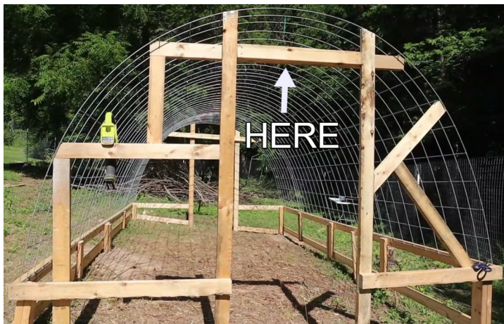
FIG 37. EXTRA 2 x 4 TO SUPPORT THE RIDGE BEAM
