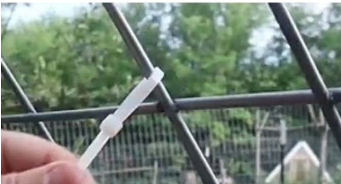
FIG 17. ATTACHING PANELS TO EACH OTHER
