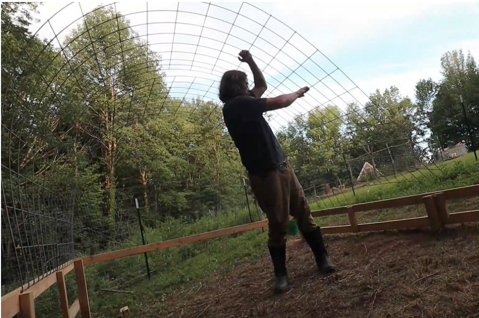
FIG 16. BENDING THE SECOND PANEL
