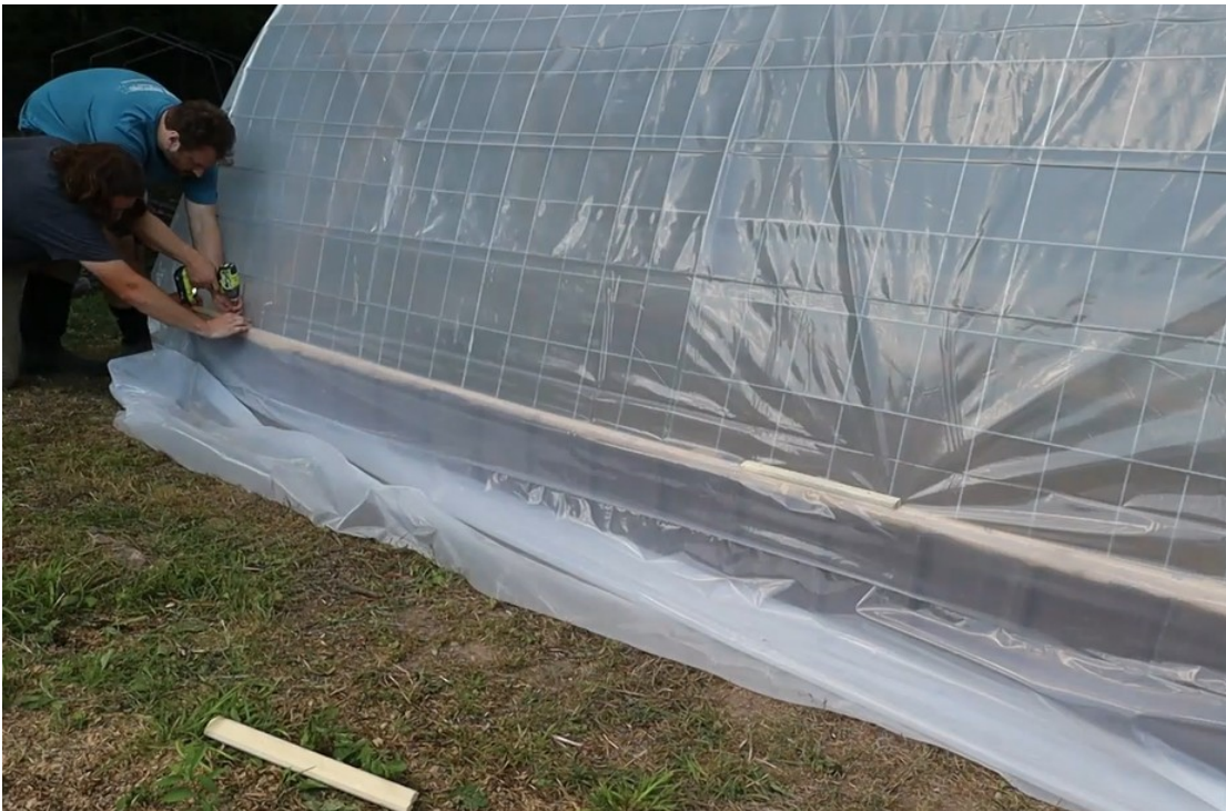
FIG 46. SECURING PLASTIC USING FURRING STRIPS
