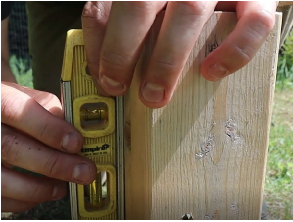
FIG 3. CHECKING ANCHOR POINTS FOR PLUMB
