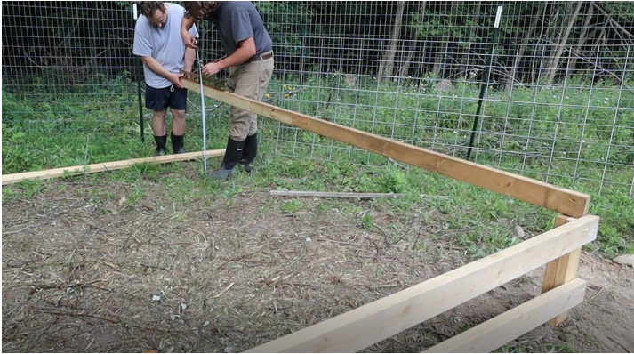
FIG 6. LEVELING END TO GET SIDEWALL HEIGHT
