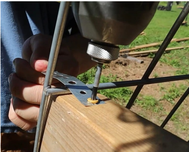
FIG 33. PLUMBERS TAPE TO ATTACH BRACING TO CATTLE PANEL
