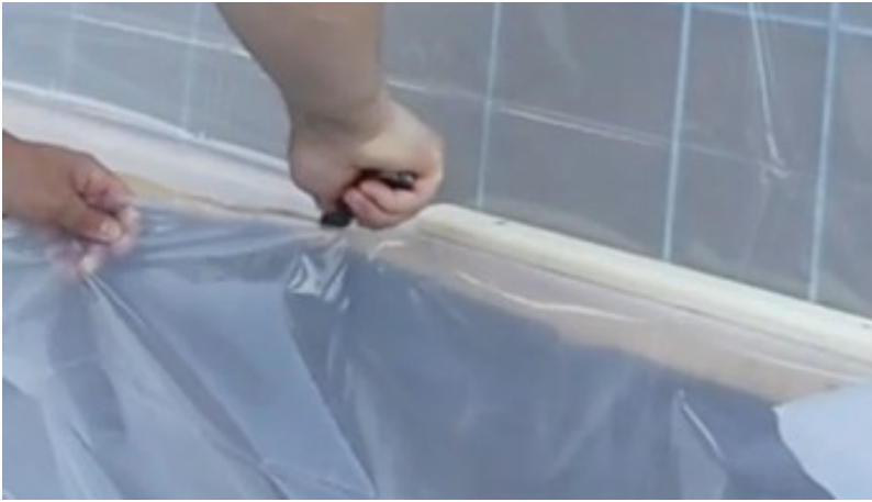
FIG 47. TRIMMING EXCESS PLASTIC
