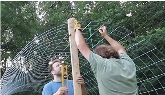
FIG 23. LINING UP CATTLE PANEL WITH MID POINT
