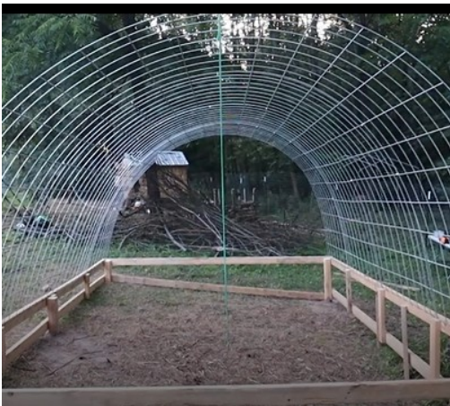
FIG 22. HANGING PLUMB BOB FROM CATTLE PANEL.
