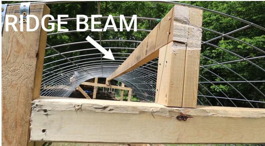
FIG 36. CONNECT THE RIDGE BEAM TO EACH SUPPORT
