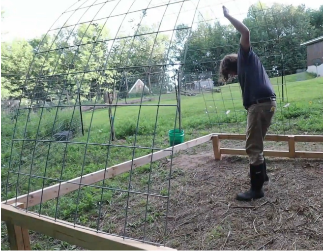
FIG 13. BENDING THE CATTLE PANELS
