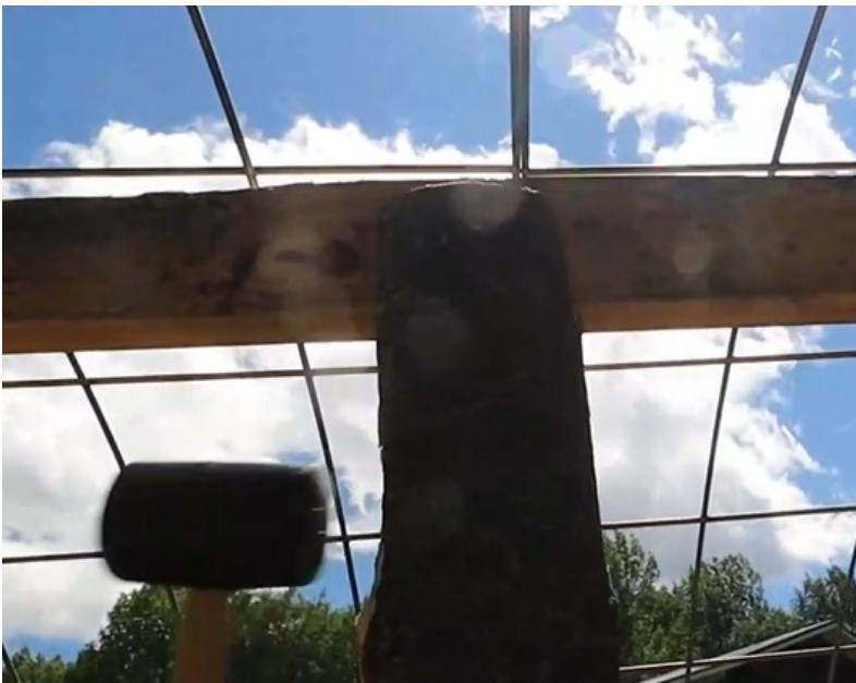
FIG 40. WEDGING SUPPORT INTO PLACE
