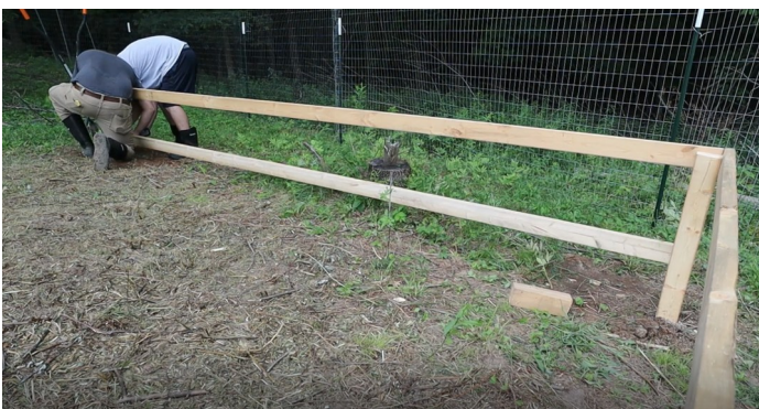
FIG 8. COMPLETING SECOND SIDE WALL
