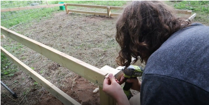
FIG 9. ATTACHING TOP CROSS BAR ON FRONT WALL
