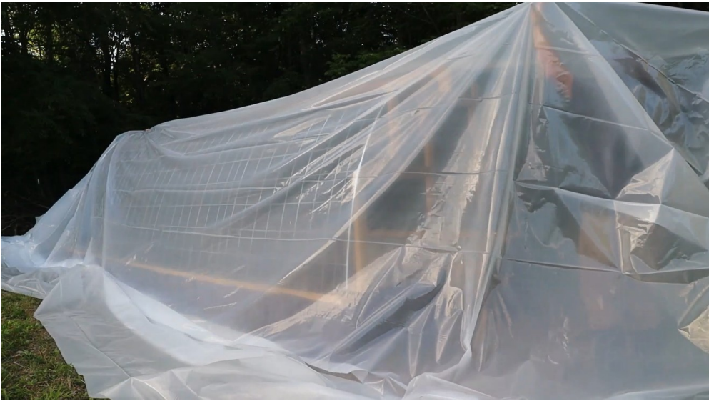
FIG 45. SLIDE PLASTIC OVER TOP
