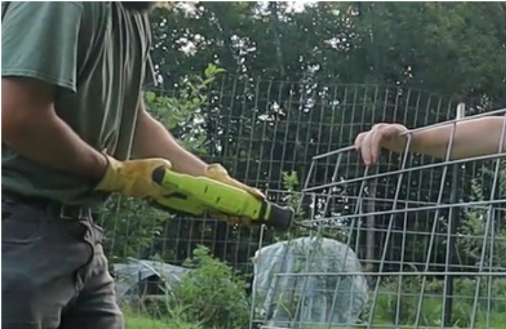
FIG 19. CUTTING THE FINAL PANEL
