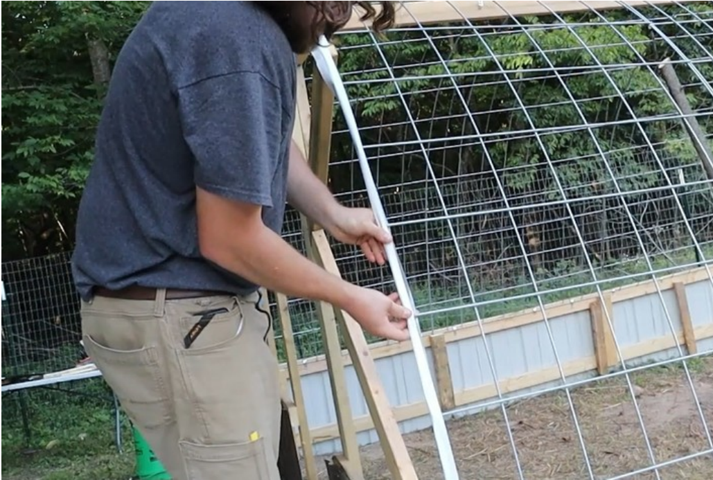
FIG 43. PROTECTING THE GREENHOUSE PLASTIC FROM THE PANEL ENDS
