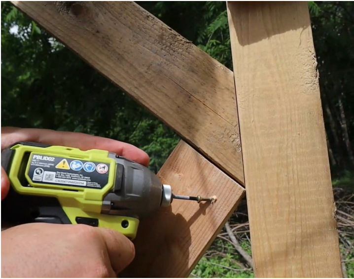
FIG 31. SECURING BRACES TO DOOR FRAME
