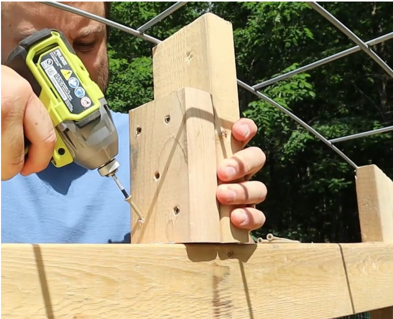
FIG 35. RIDGE BEAM SUPPORTS ON EACH HEADER
