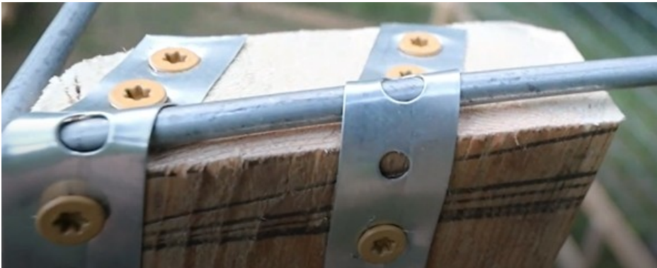
FIG 25. SECURING DOOR-FRAME TO CATTLE PANEL
