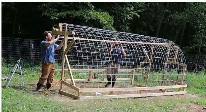
FIG 38. RAISING THE RIDGE BEAM
