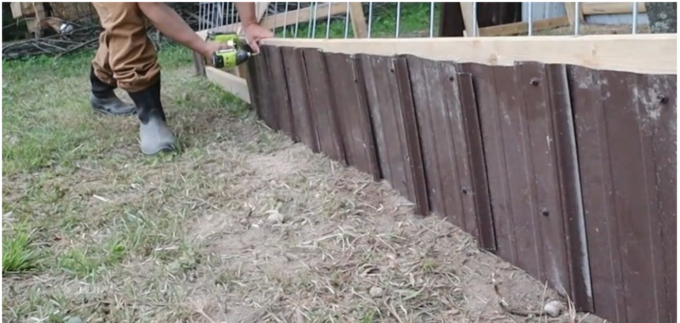
FIG 42. MORE METAL WORK
