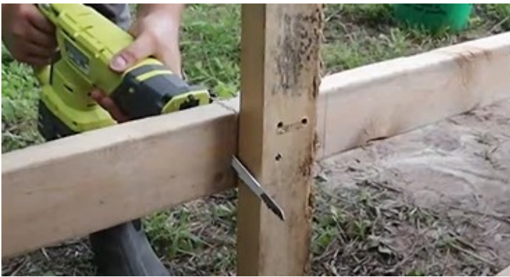
FIG 27. CUT OUT CROSS BARS
