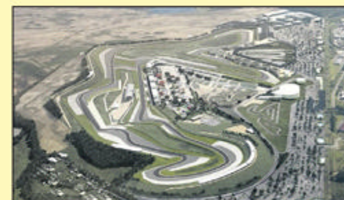
Building Circuit of Wales was to start this week
