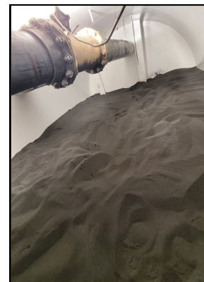
Above: The exterior of a pressure filter is shown. At left: A layer of filter media is shown in the interior of the pressure filter.
