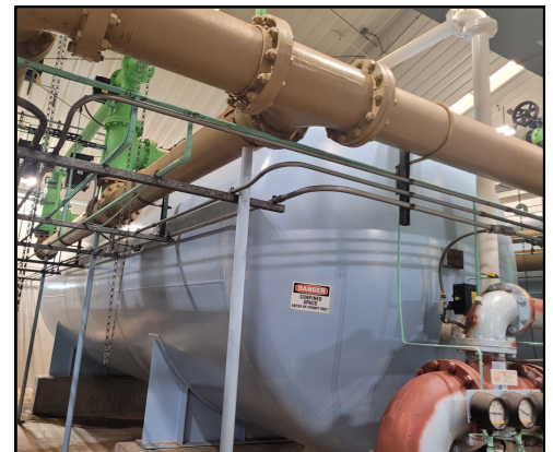
Above: The exterior of a pressure filter is shown. At left: A layer of filter media is shown in the interior of the pressure filter.
