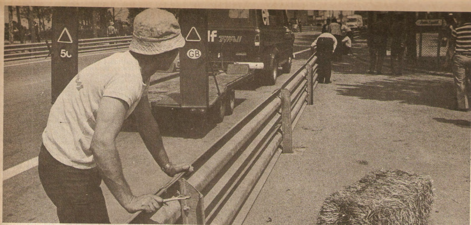
The constructors turned Armo erectors . . .
