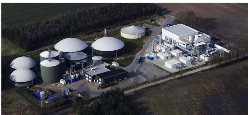
Fig. 13. Audi e-gas plant (source: EWE).
