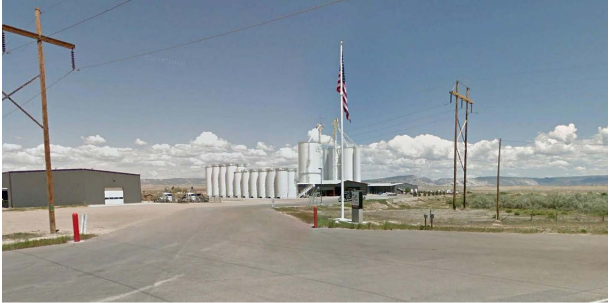
Figure 8 - The Goodrich Mud Company terminal in Vernal, UT.
