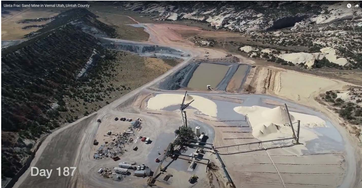
Figure 4 - Processing plant at the RHEX plant in Vernal, UT.
