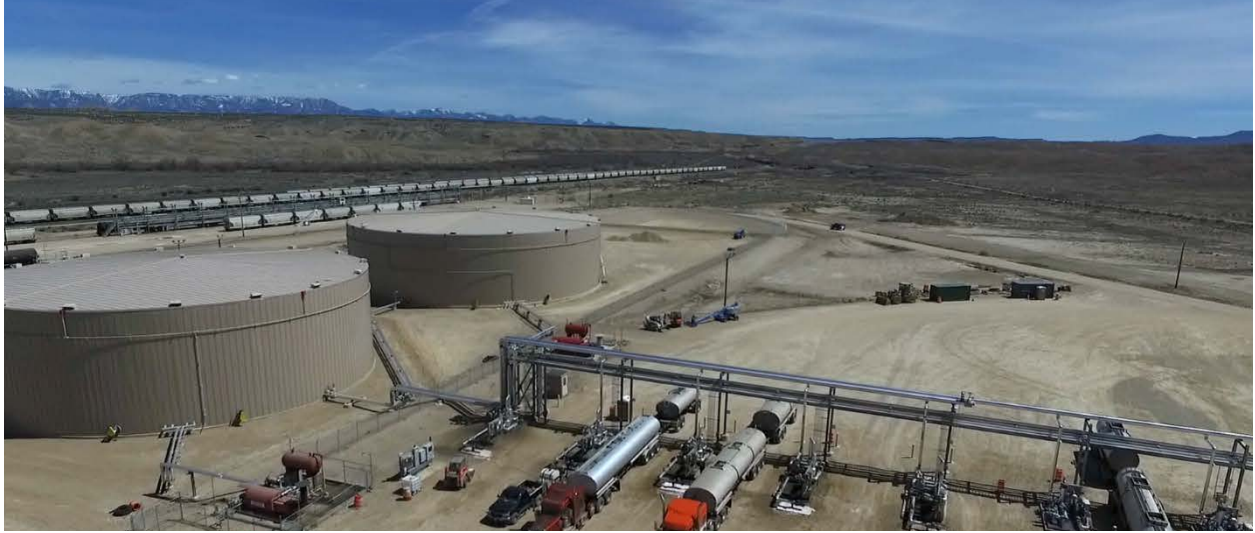
Figure 6 - Price River Terminal Transloading facility.
