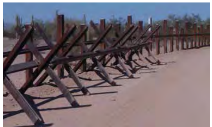
33 Mile Vehicle Barrier
