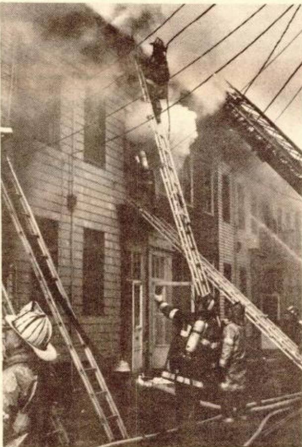
FIRE FIGHTERS at the six alarm fire on Wall Street battle the blaze in heavy smoke and among a web of low-hanging wires.
