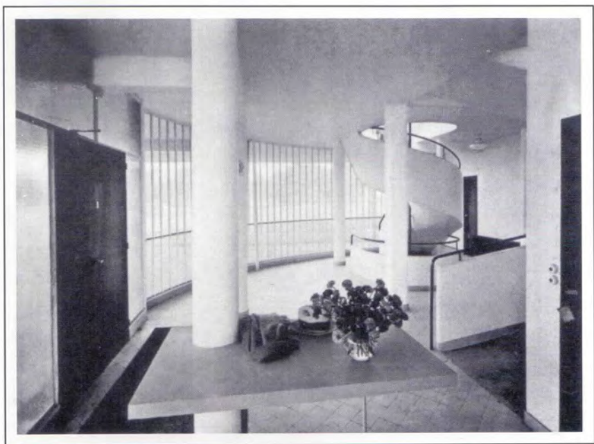
Villa Savoye. The entrance hall.
