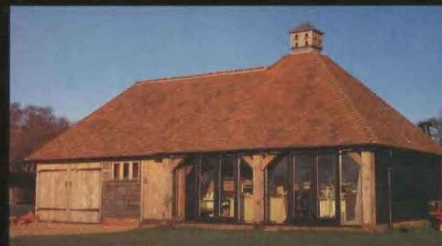
GARAGE & OFFICE COMPLEX No. 380
