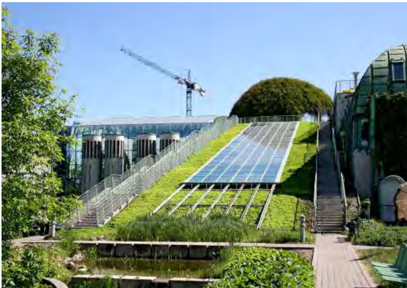
Ecological modern building . Warsaw University in Poland.
