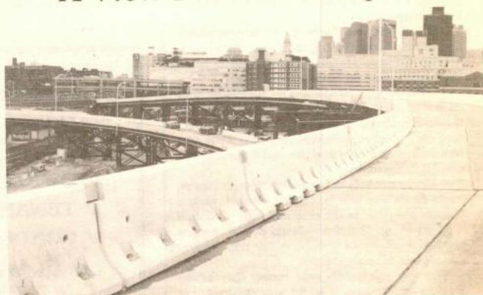
THE TWO-TIER temporary ramp structure carrying traffic to and from the Tobin Bridge through the newly constructed tunnels under City Square is set to open. The northbound ramp has been scheduled to open today, Sept. 1, with the southbound ramp due to open on Sept. 8. According to the Mass. Highway Department, demolition on the overhead structure in City Square will begin a week after the opening of the second ramp, starting at Gate 1 of the Charlestown Navy Yard, and work will proceed toward Route 93 with the completion of Chelsea Street before winter.
