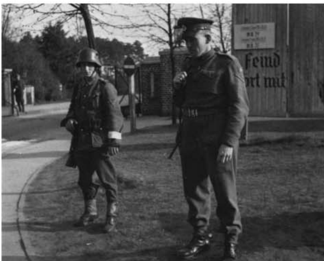
The barracks was garrisoned by some 800 German and 3,000 Hungarian troops (Hungary was allied to Germany and Bergen was also the training school for the Hungarian Army armoured corps). Under the truce, the garrison was allowed to retain its arms, the Hungarians remaining at the disposal of the British
