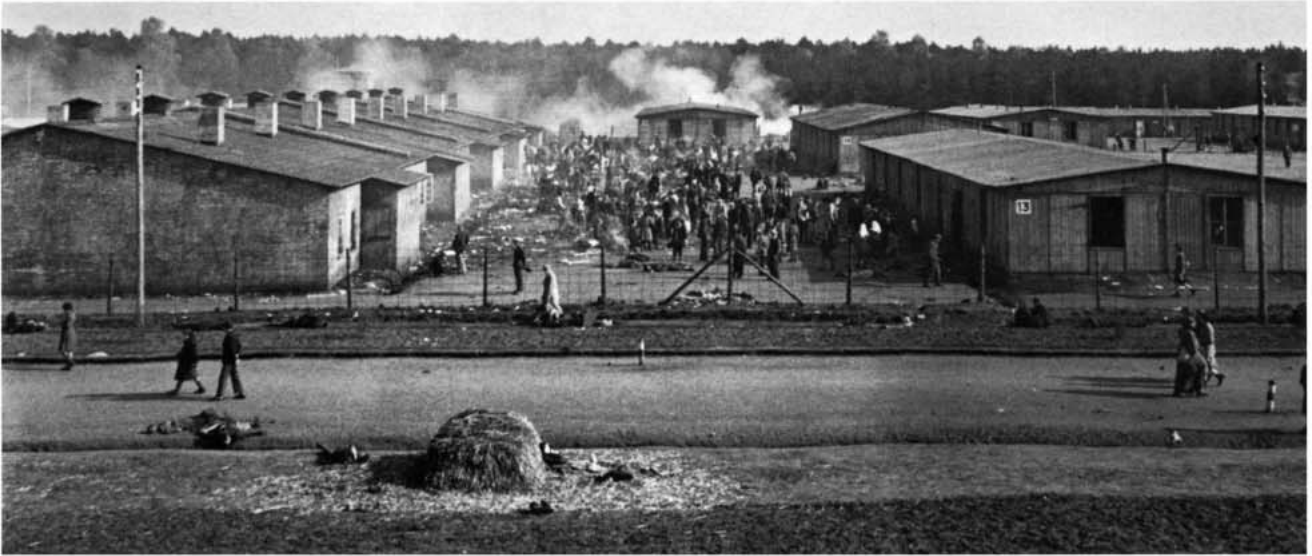
At the camp itself, Huts 11 (left) and 13 originally belonged to different sections of the camp, No. 11 being one of the two huts of the Hungarians' Camp and No. 13 being one of those erected in the Star Camp after September 1944. However, by 1945, the last of the Hungarian Jews had been exchanged to Switzerland, and the ever-expanding Prisoners' Camp had
