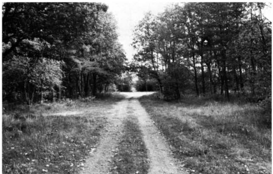
The same view today. Once the gate to 'hell on earth', now just a track leading into the woods. Nothing — not even a trace of its foundation — remains of the guard-house on the right.
