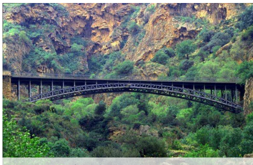
Pont Eiffel Tlemcen
