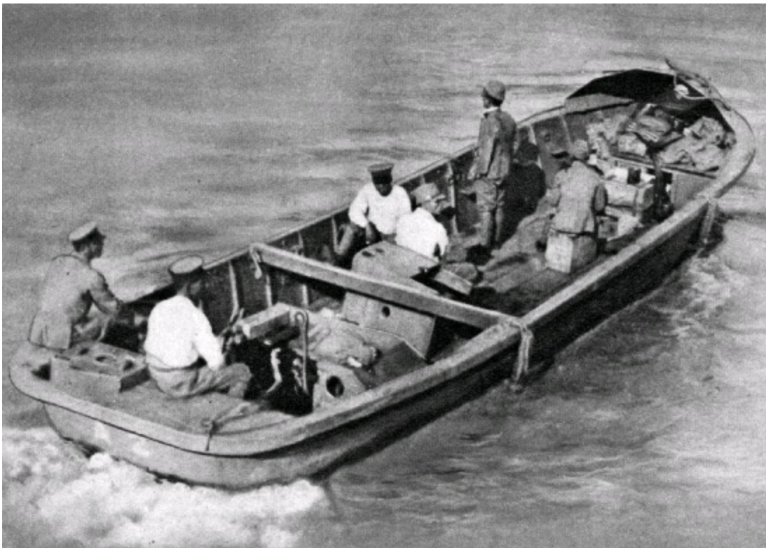
The Type F Japanese barge was designed as a small personnel carrier. At a length of twenty-one feet and with a beam of seven feet, it could carry approximately twenty men. It was not armed and the crossbeam could be moved to shift compartment arrangements. U.S. War and
