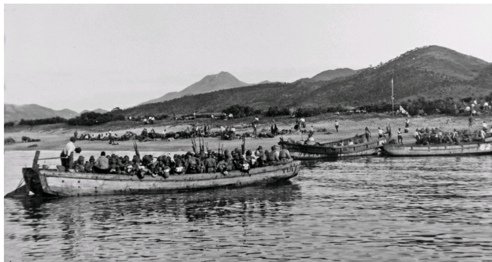
A Japanese Type D barge lands troops near Canton, China, on 12 October 1938. This type of barge was built in several variations ranging from 38 feet to 70 feet. NARA 306-NT-1151-J-4.
