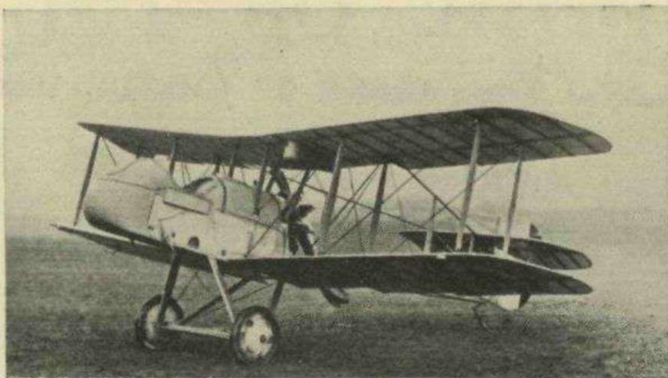
A famous D.H. aircraft and an ancestor of the "Moth"—the D.H. 2 "pusher" scout of 1915-1916.
