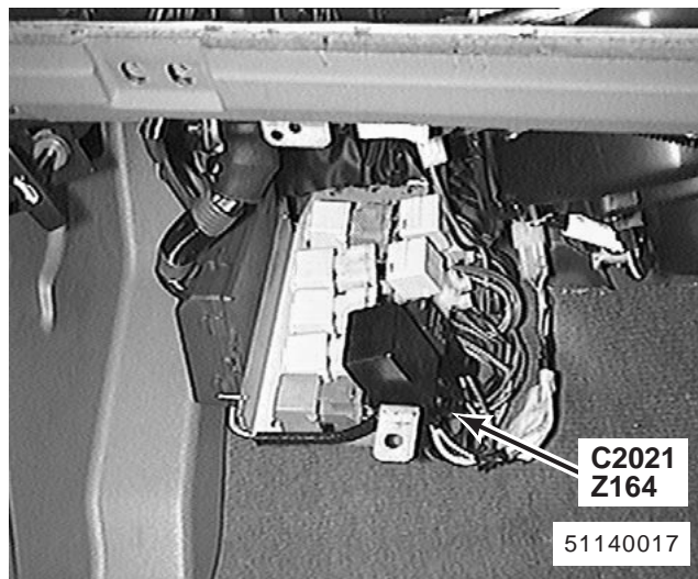
234. behind LH side of fascia (Manual Transmission) Z164 Speed Trip Module C2021 (5-B)
