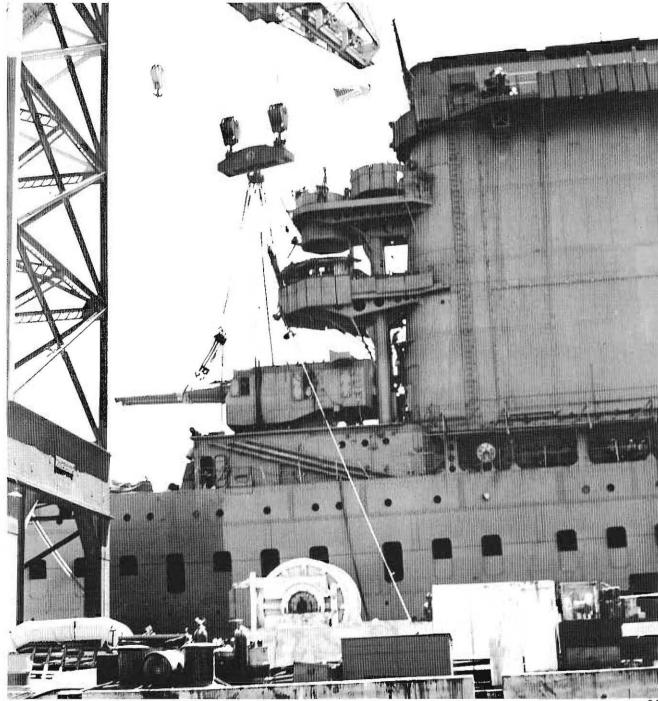
This close-up view of turret #3, as it was lifted into the air from the superstructure of LEXINGTON, shows the multitude of rivets used in the construction of this type of gun mount.
