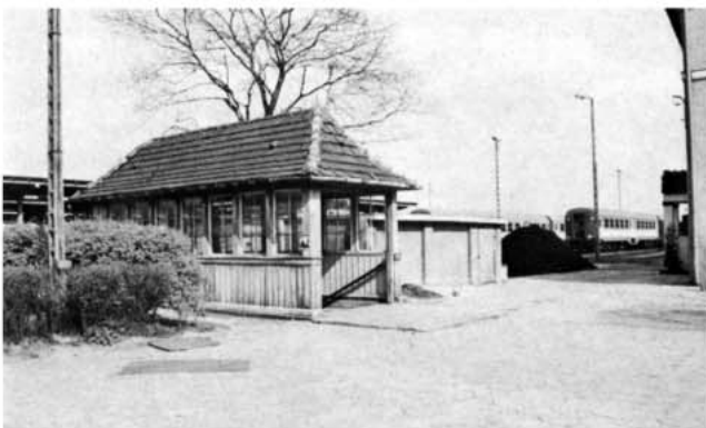
Although the main entrance lay north of the line, the prisoners knew that a rear entrance (left) led via a subway under the tracks to the booking hall (right). However, the subway was protected by a storm porch and, in the darkness, most of the
