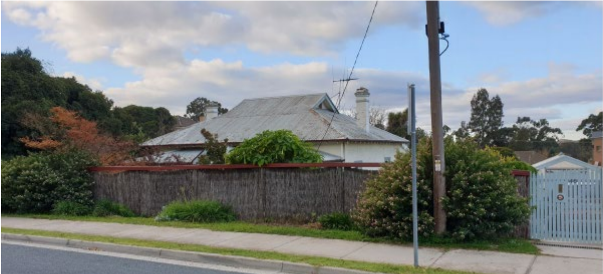
Figure 6: Existing dwelling at 48 Nolan Street
