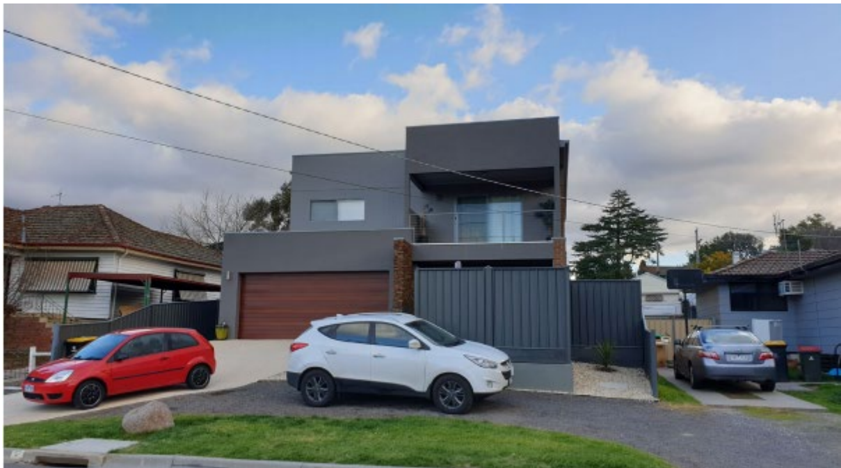
Figure 7: Existing dwelling at 5 Dooley Street
