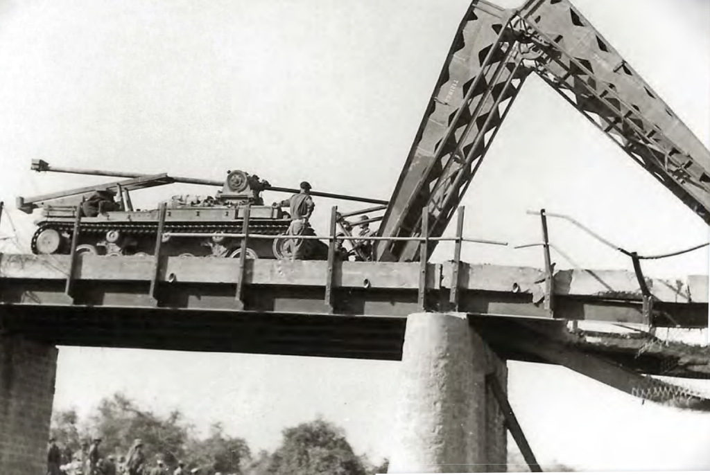
Above: T16278 is now in the Tank Museum. Here it is seen being inspected by two young soldiers. There were no markings on it when this photo was taken. Left: A Valentine scissor bridgelayer emplacing its bridge over a broken bridge in Burma.
