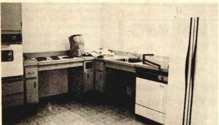
THE FIRST FLOOR APARTMENTS are reserved for handicap residents. Notice the stove and sink are placed low with plenty of leg room underneath for easy access to wheelchair persons.
