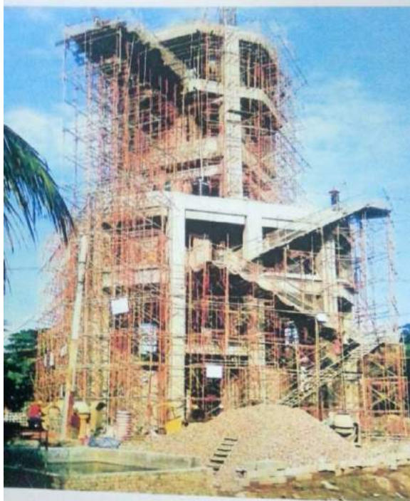
Construction Work Start – 2008
