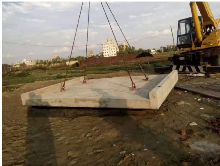
Precast Slab Lifting Shifting
