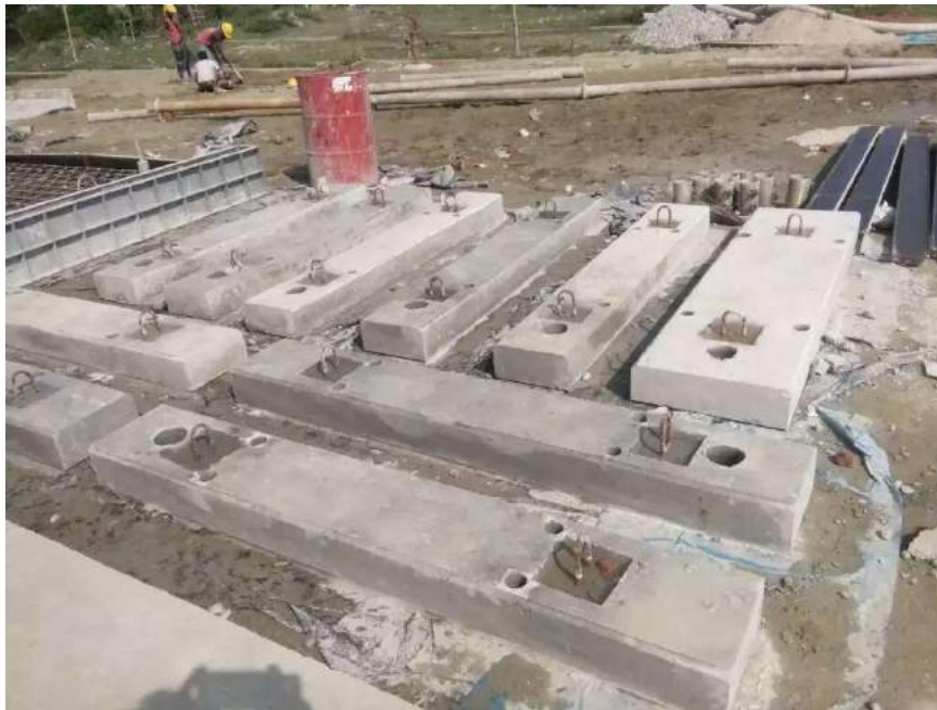
Precast Slab Casting Work
