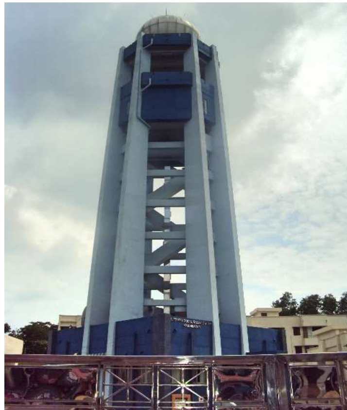
Complete Project – March, 2010
