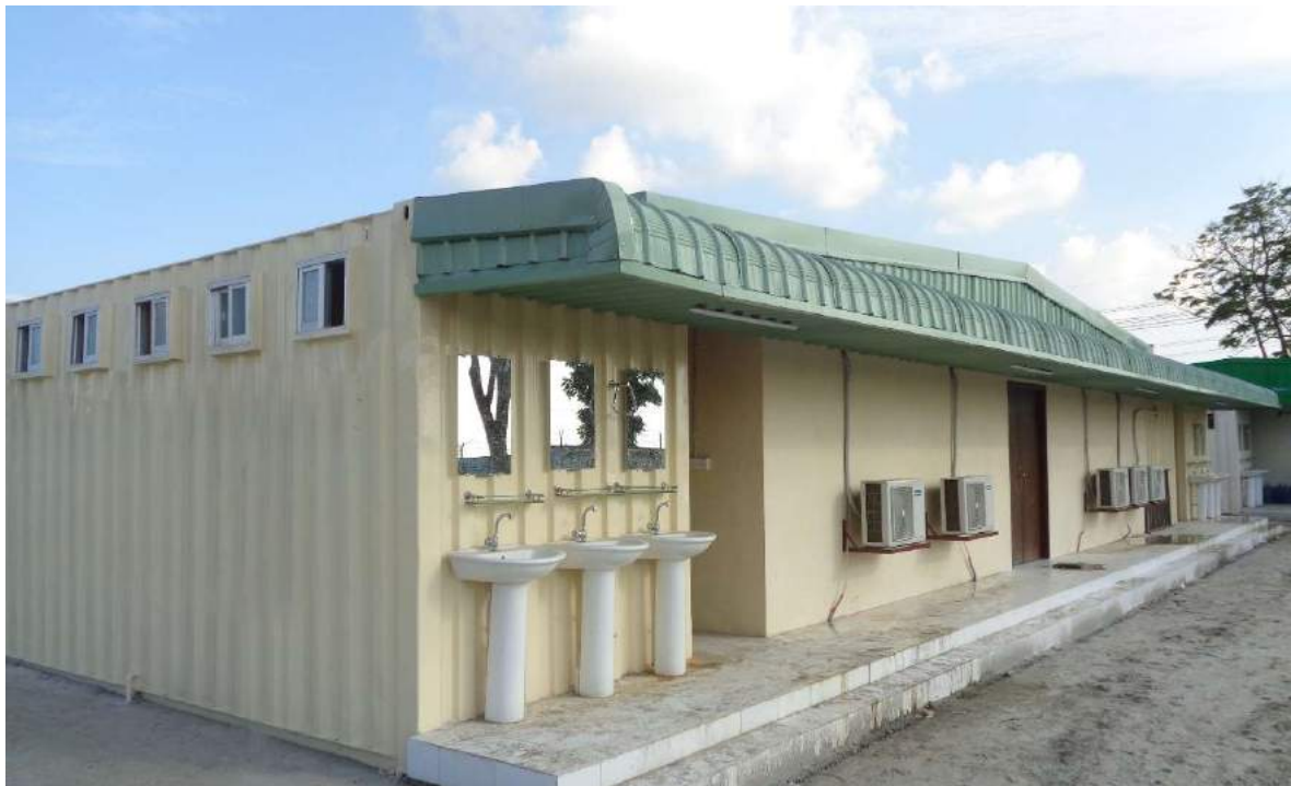
3 nos Complete Police Accommodation -2016-17
