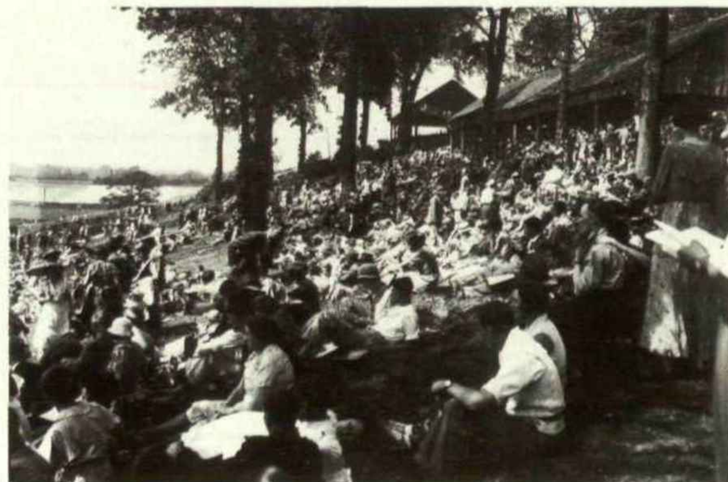
Below the Members' Hill tea-rooms, looking over the Test Hill
