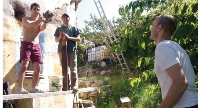
6/13: West wall: Building the porch / Pared oeste: construir el porche
