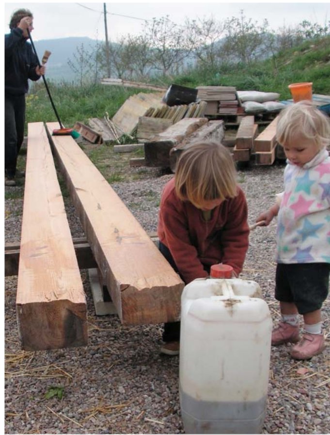
4/08: Treating beams with linseed oil / Tratando vigas con aceite de linaza
