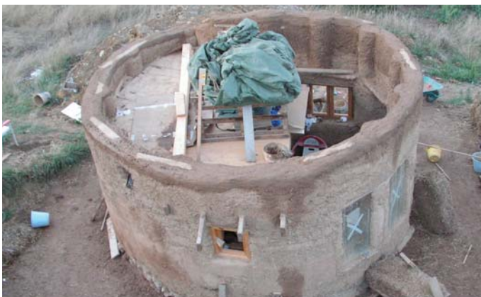
7/06: The wall finished / El muro terminado
