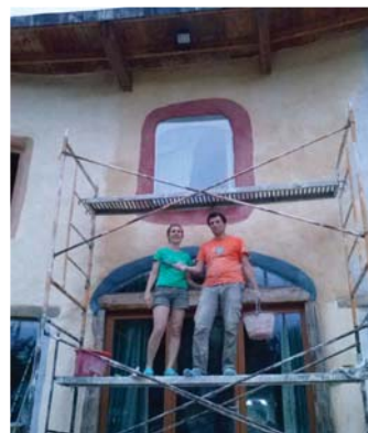
10/13: Painting house front / Pintar fachada
