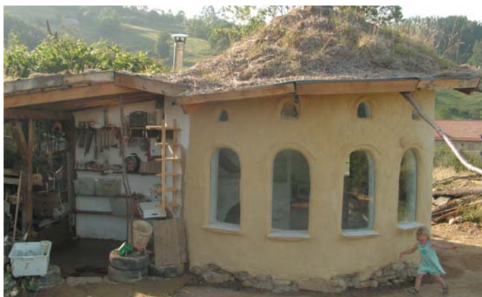
7/07: Exterior finished... well, part of it / Exterior terminado... en parte
