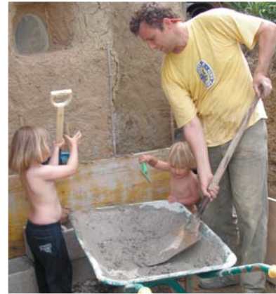
5/08: Composting toilet / Aseo seco
