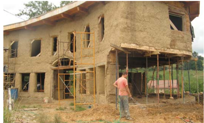
Mixing cob / Mezclando cob
