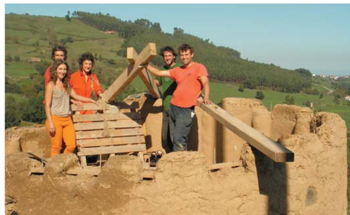
10/06: Building the reciprocal frame roof / Construyendo el tejado reciproco
