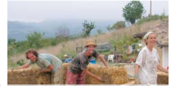
3: Applying slip / Aplicando barbotina
