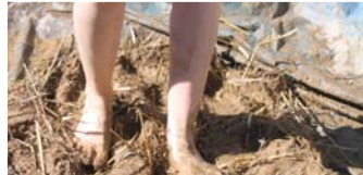
Mixing cob / Mezclando cob
