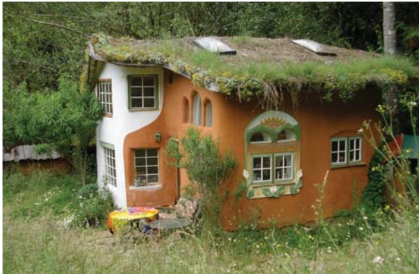
New cob houses / Casas nuevas de cob 1: Coquille, OR, USA (Cob Cottage Company)
