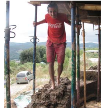
Treading the cob / Pisando el cob
