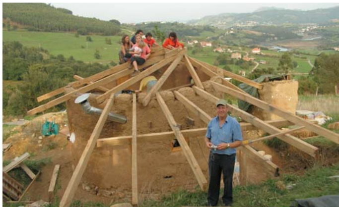
10/06: Green oak roof beams in place / Vigas de roble verde colocadas
