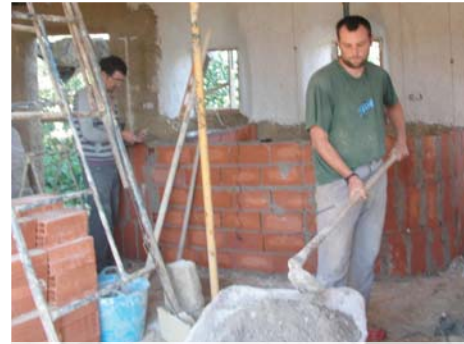
9/11: Interior brick walls / Paredes interiores de ladrillo
