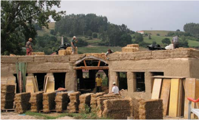
1: Straw bales prepared with slip drying / Balas de paja preparadas con barbotina secando
