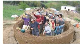
Compacting subfloor/Compactando subsuelo
