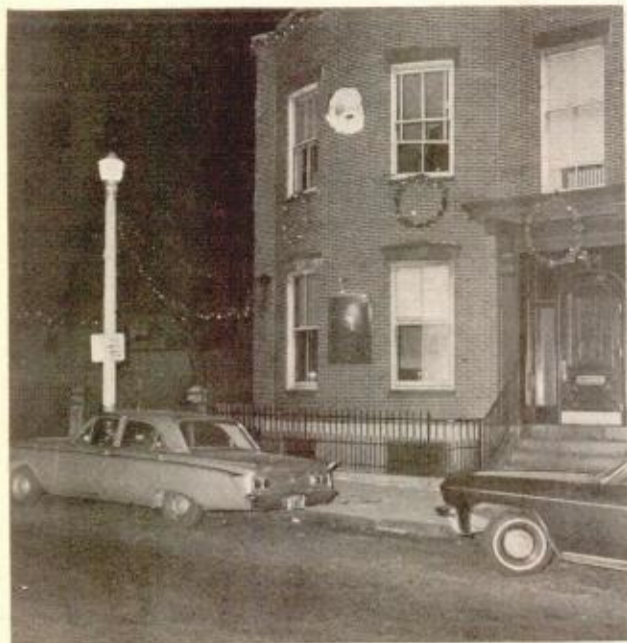
THE QUARTERS of Bunker Hill Council at 44 High Street served the members for many years. The council was decorated for Christmas in this mid-1960s photograph.
