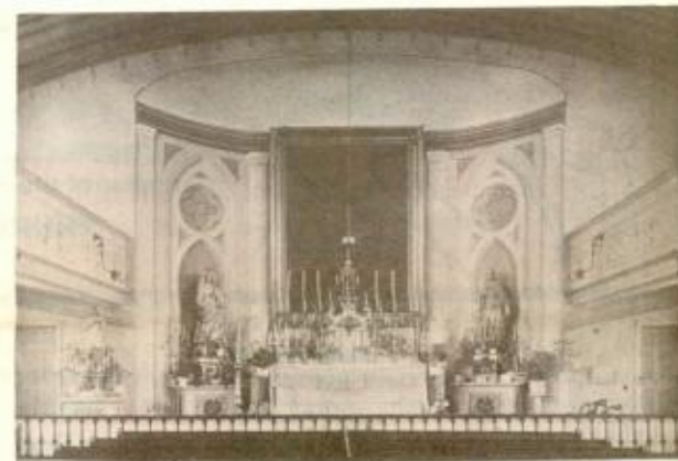
ALTAR and sanctuary of St. Mary's Church on Richmond Street where construction began in 1828. (photo courtesy of the Charlestown Branch Library)
