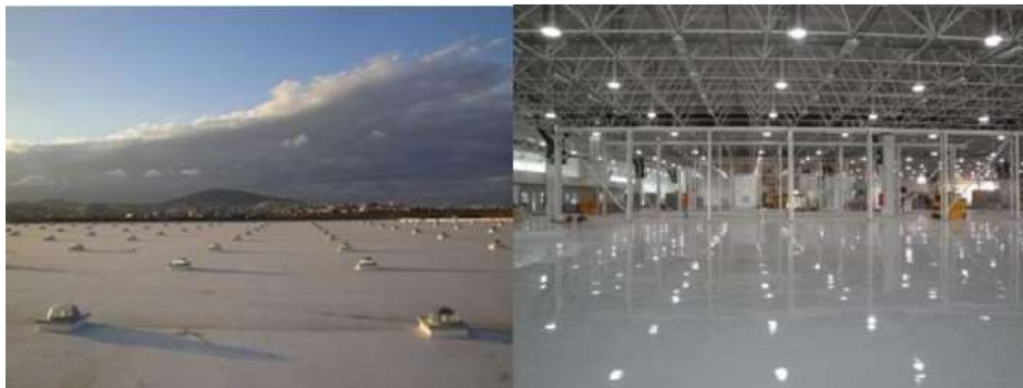
Figure 1: Light-colored membranes on the roof and building lighting [8].
