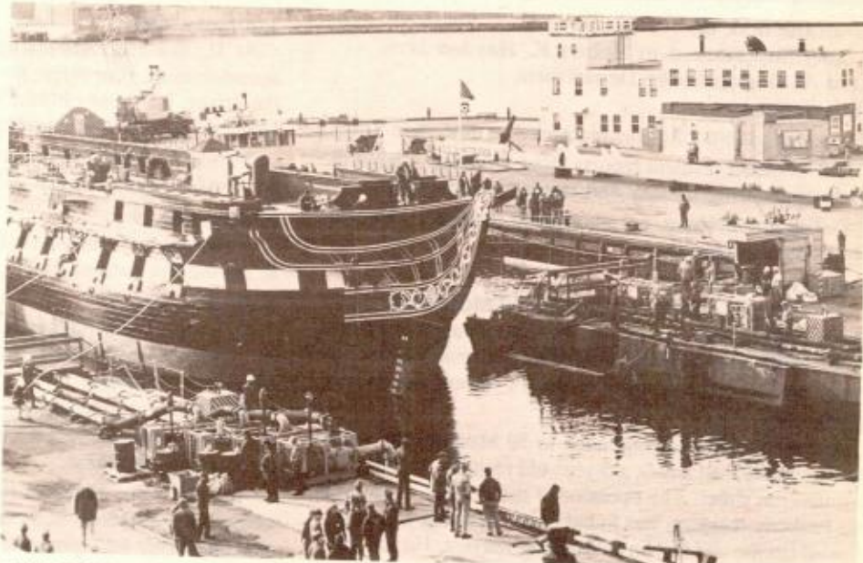
USS CONSTITUTION crossing the sill of Dry Dock 1, Boston National Historical Park, Charlestown Navy Yard on Sept. 25. The 194-year-old frigate will be inspected and repaired in the dry dock, a procedure that is expected to be accomplished over the next 12 months, in preparation for her bicentennial in 1997. (photo by Tom Hannon, Constitution Joint Information Bureau)
