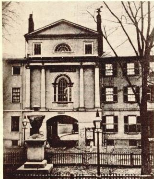
THE PAVILION CENTER of Bullfinch's famous Tontine Crescent Building is shown above in this reproduction of an old photograph. A similar reconstruction of the Pavilion can be seen in the Kirstein Business Library behind Old City Hall.
