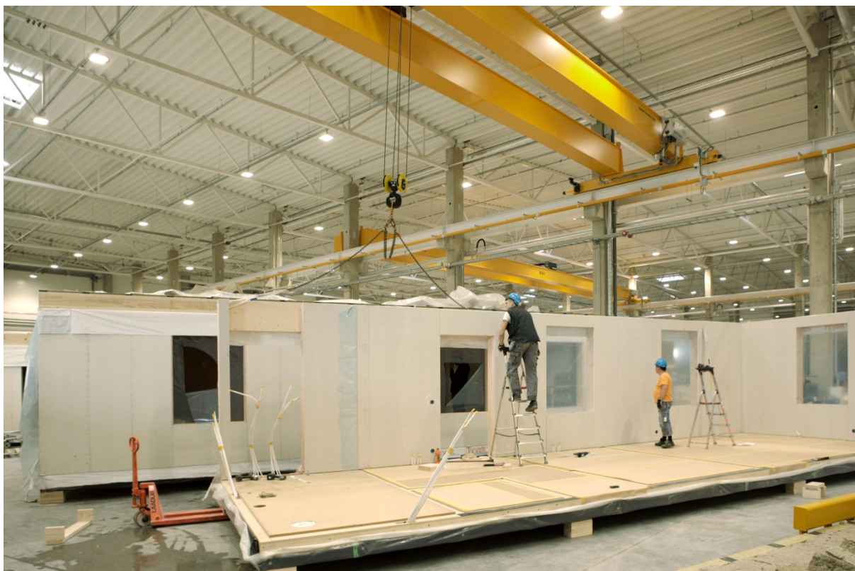
Figure 13. Example of a 3D-assembly phase at Harmet's (courtesy of Harmet).
