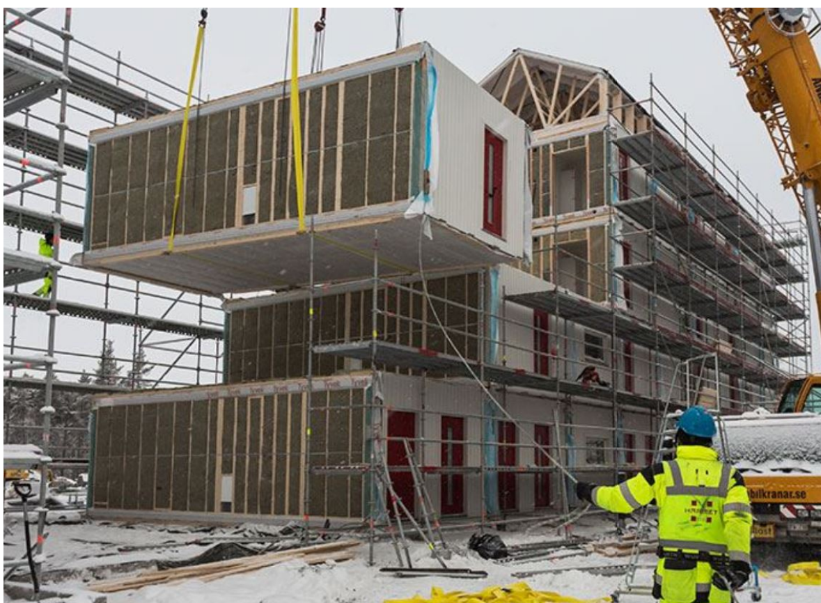
Figure 17. Construction of a modular wooden house (courtesy of Harmet).
