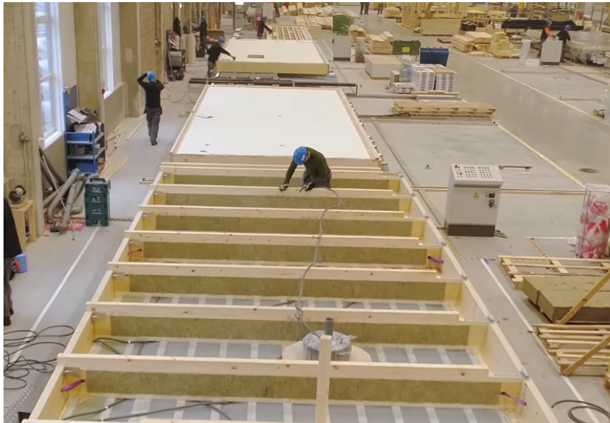
Figure 12. Example of a 2D-assembly phase at Harmet's (courtesy of Harmet).
