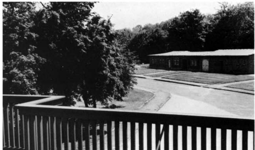
The field-guns have long gone but the SS building still survives, albeit with post-war extensions. Picture taken from the balcony of the main gatehouse seen overleaf.
